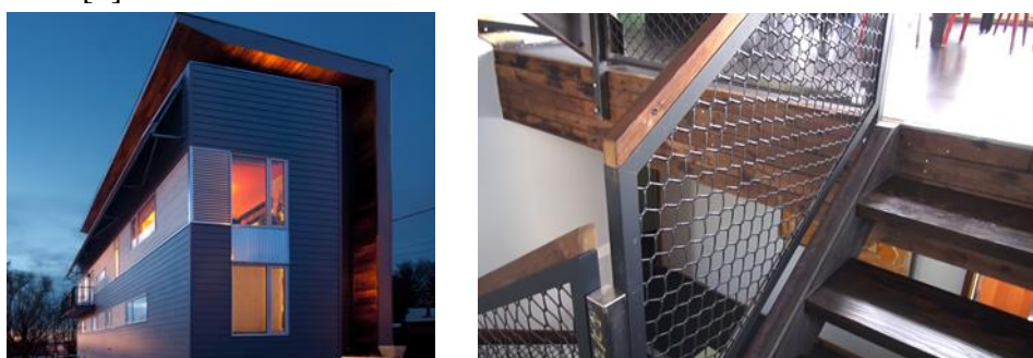
Figure (2). Shafraaz and Serena Kaba net-zero home. By Shafraaz, Canada Best users for fully zero energy home – using extra structure materials in stair construction http://www.greenenergyfutures.ca/episode/episode-80-chasing-net-zero-net-zero-evolution
