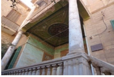
Pl.3: The Middle Part of the Northern Façade (By the Researcher)
