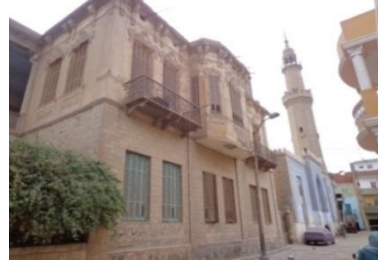
Pl.4: The Western Facade of Abd Al-Azim Abu El-Nil's house (By the Researcher)
