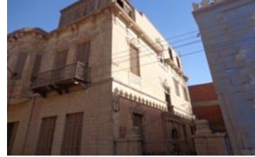
Pl.6: The Southern Facade of Abd Al-Azim Abu El-Nil's house (By the Researcher)
