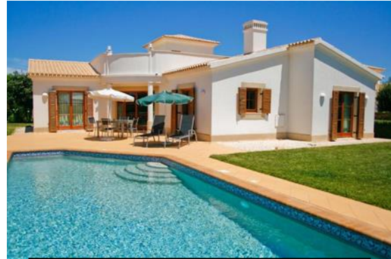
FIG.7, External doors and windows
