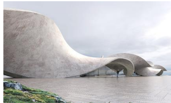
FIGURE 20. THE TWISTED SCULPTURE-LIKE CONCRETE HOUSE BY ANTONY GIBBON, ALIGNED THROUGH THE LANDSCAPE
