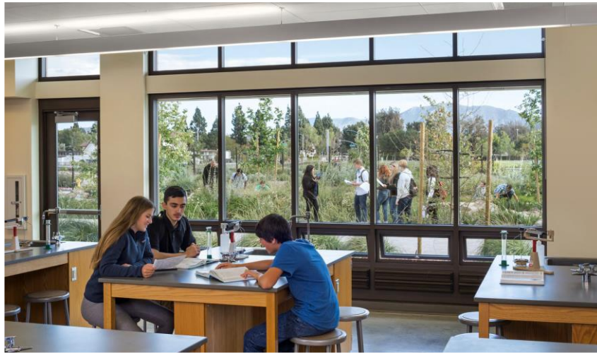
Figure ( 5 ) illustrates using of sustainability principles to design natural ventilation strategies, operable shade windows and night vents - control of water flow - drainage. Oxnard Union County Rancho Campana High School (Designed by HMC Architects)
