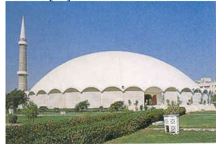
Karachi: The use of concrete shell dome to cover the whole prayer area of Defence Officers' mosque [10]
