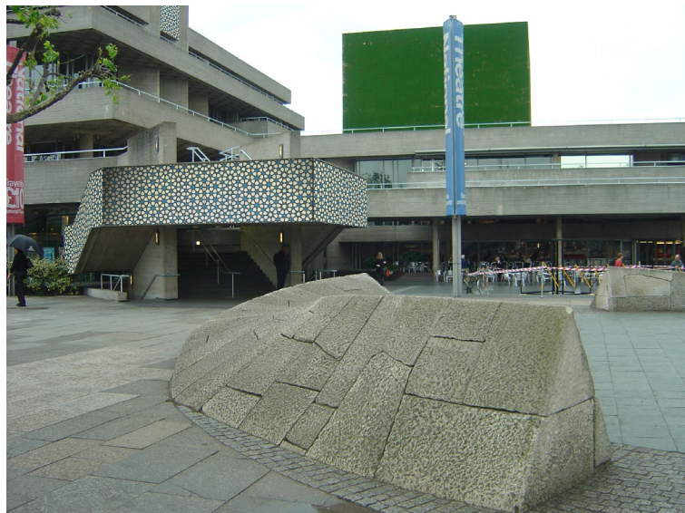
Figure No.18 Detailed picture for the same design, from a different angle
