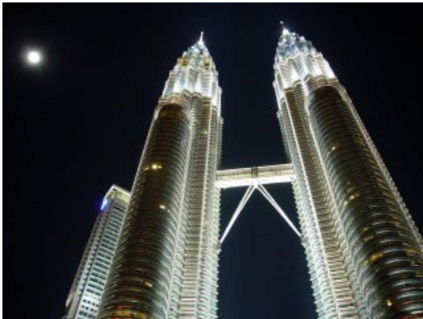
Figure No.9 Petrons twinTower, Malaysia 1998.
