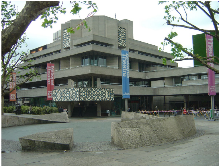
Figure No.17 A hypothetical design made by the author for the National Theatre building in London, UK 2007 Projection art
