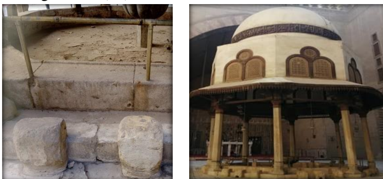
Ablution Unit and place to sit in front of each faucet - Sultan Hassan Mosque - Al-Qalbaa Figure (11)
