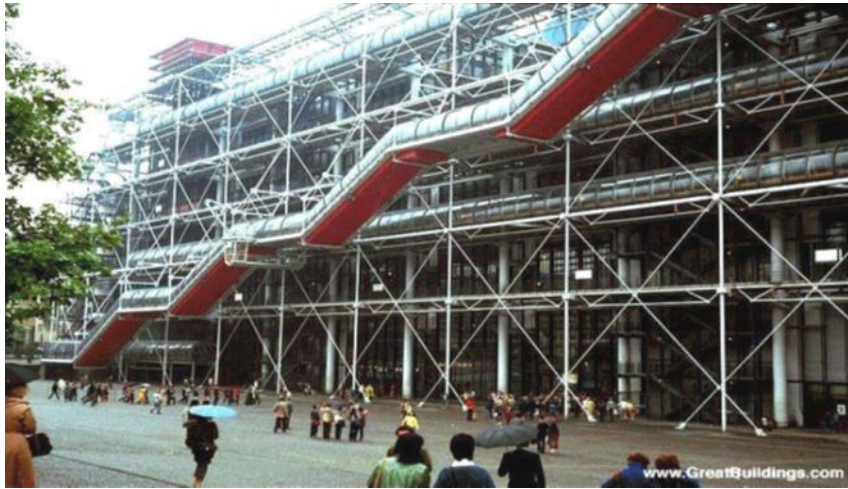
Fig (6) shows the effect of technology on construction in the architectural formation of the buildings of Pompidou cultural center- Paris-France. Designed by the architects (Rogers and Piano)
