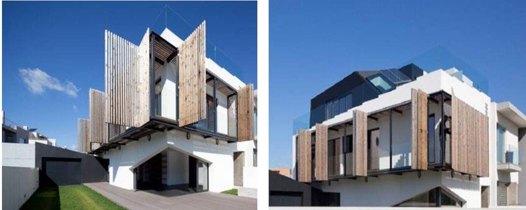
Fig (14) architectural formation at a private house using Mashrabiya (bay).
